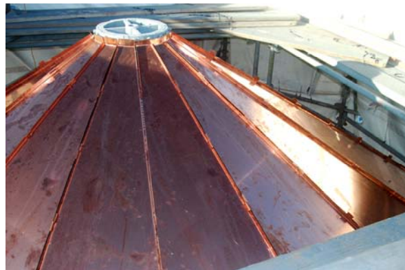
new lighthouse copper roof (Nik Epanchin)
